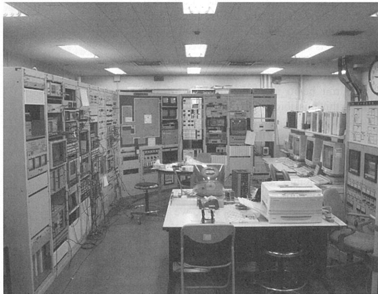
Control Room of UVSOR
