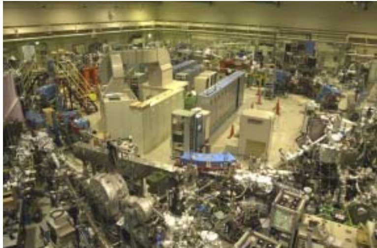
FIGURE 3. UVSOR just after removing old accelerator components
