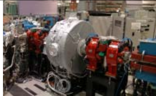
Fig. 3 Photograph of new cavity covered with jacket heaters. A view from outside the storage ring.
