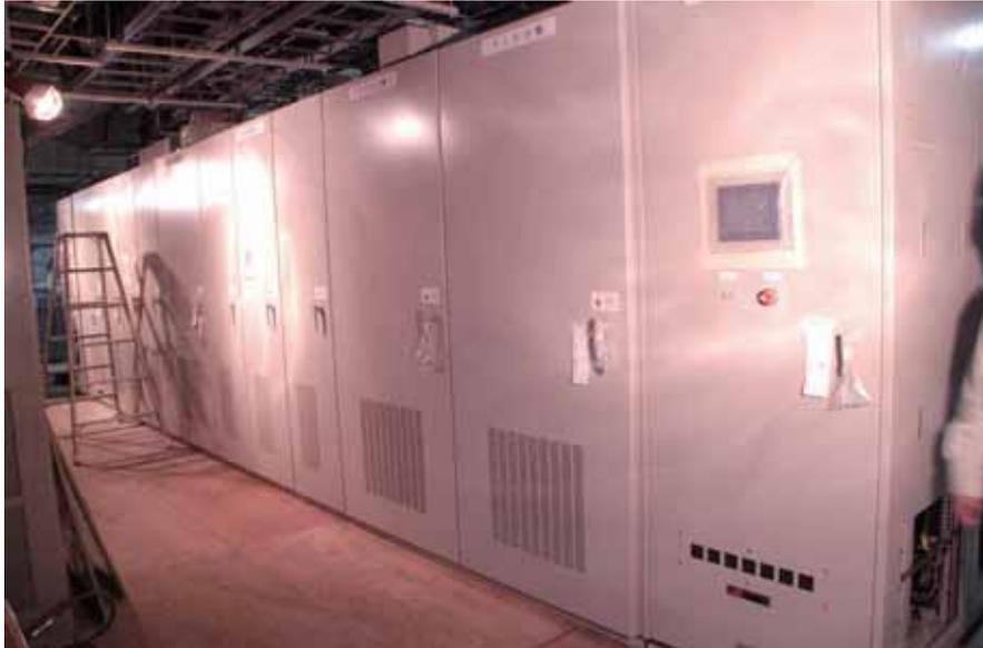
Figure 2 New Magnet Power Supplies for Booster Synchrotron
