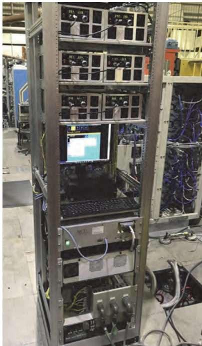
Fig. 4. New Control system for the undulator U6
